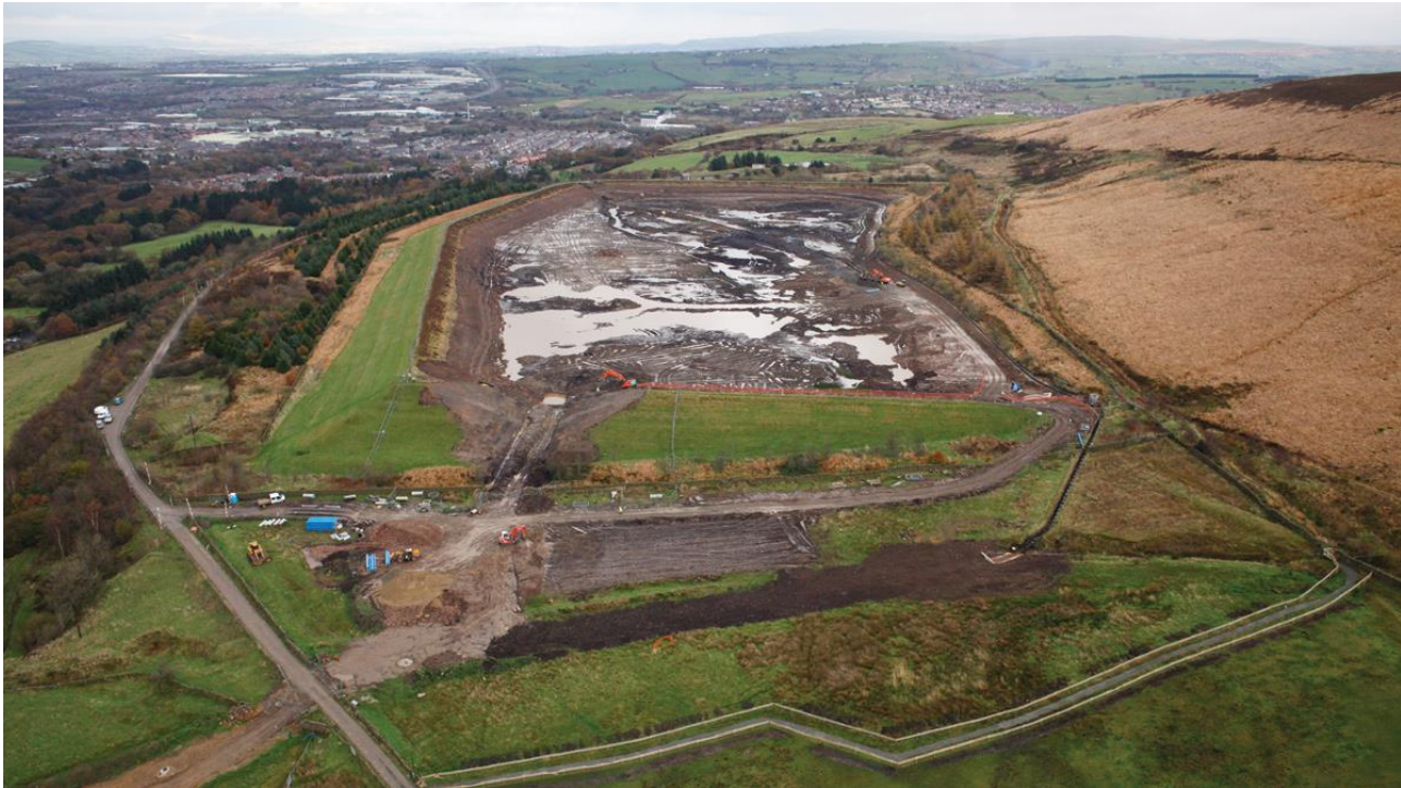
Figure 2: Sunnyhurst notch during construction - Courtesy of Suave Aerial Photos 2
