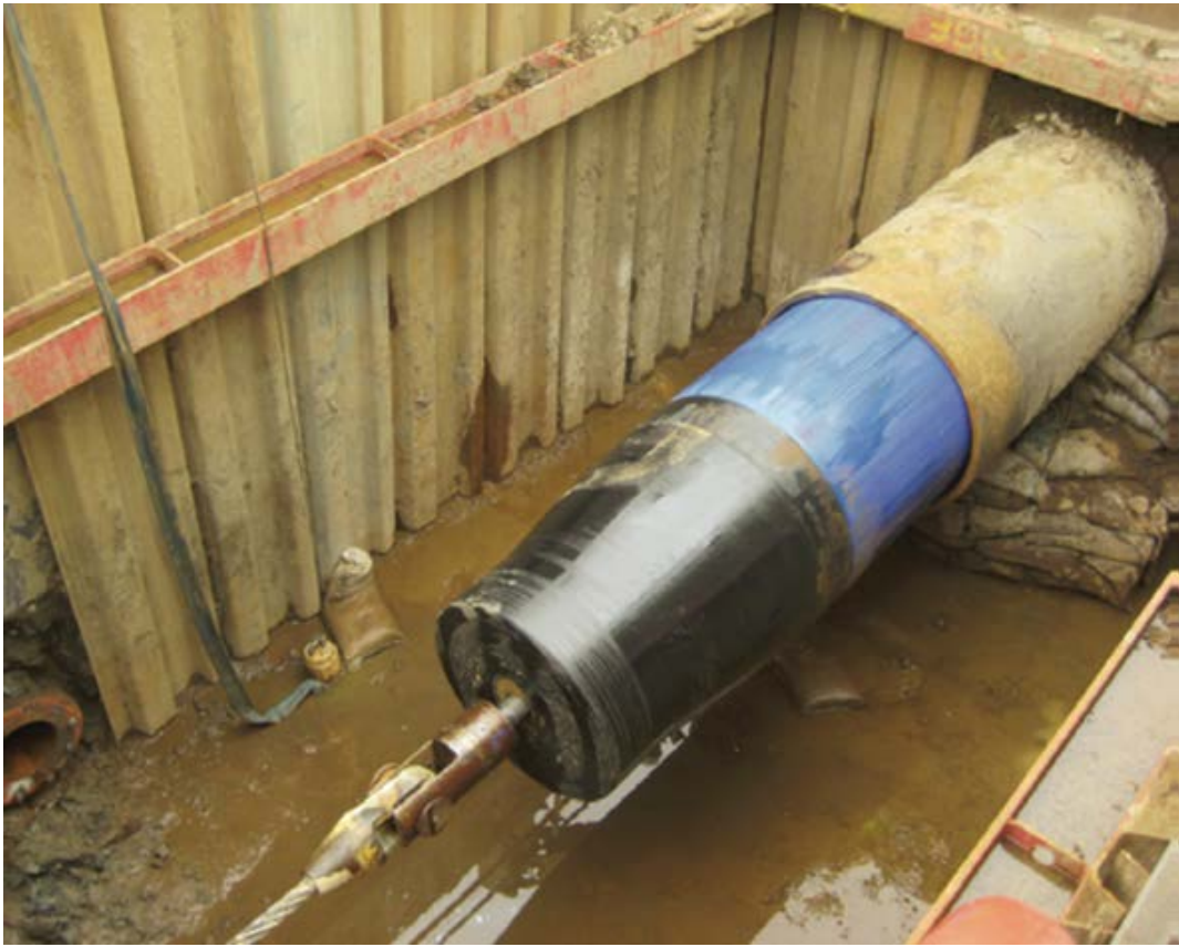
iv. Photo of pipe being pulled into host pipe
