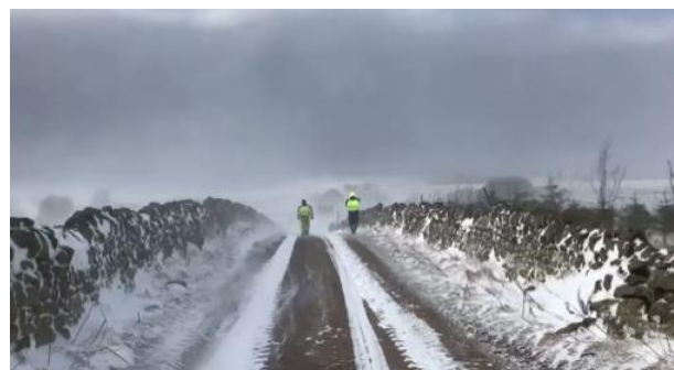
Figure 18: Challenging access conditions in the freeze (March 2018)
