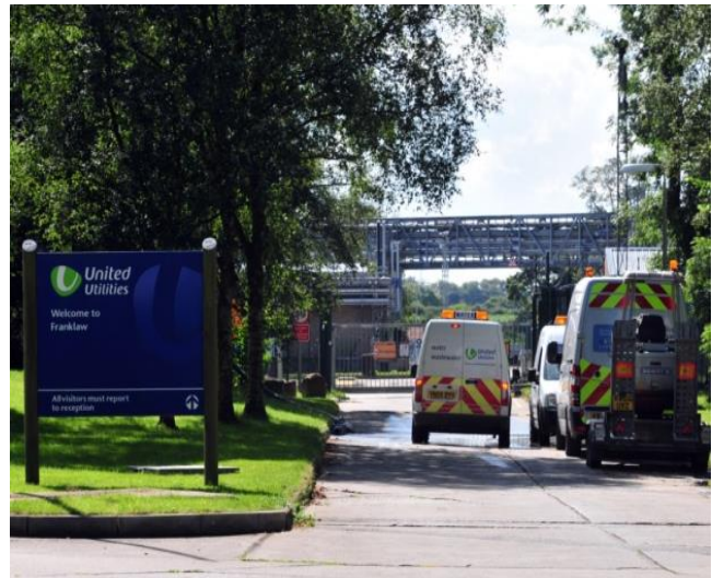
Figure 11: Franklaw Water Treatment Works
