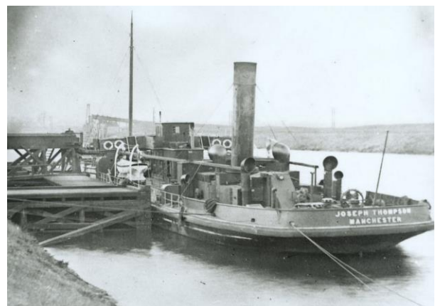
Figure 6: Sludge vessel being loaded in 1898 - featured in the Manchester Evening News
