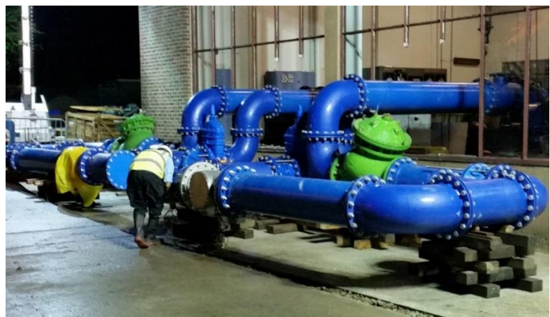
Figure 14: Installing UV treatment during the Franklaw incident
