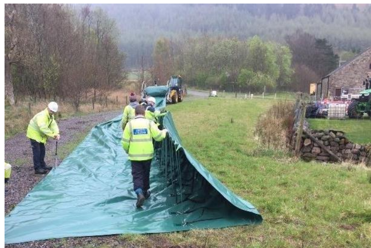
Figure 17: Temporary flood barrier being deployed in-situ at Ennerdale Water Treatment Works
