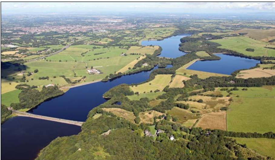
Figure 22: We are improving the asset health of our 165 impounding reservoirs
