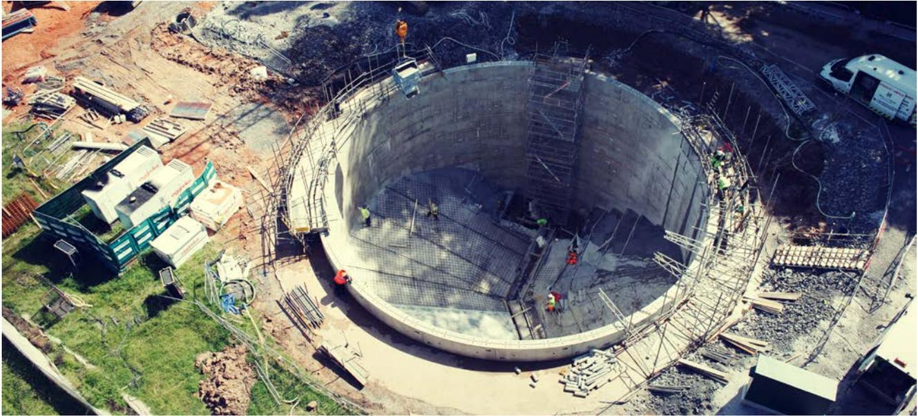
**Pictured:** Construction of a storm tank as part of a £5 million sewer improvement scheme in St Helens. Underground tanks such as this help to store huge amounts of water during heavy rainfall, preventing flooding.
