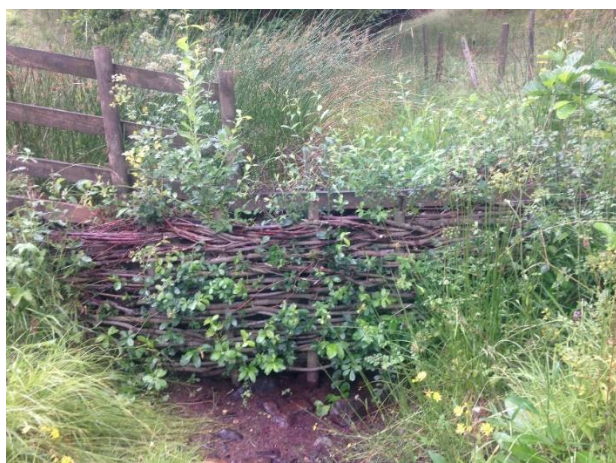
Figure 22 Physical measures – Examples of leaky dams
