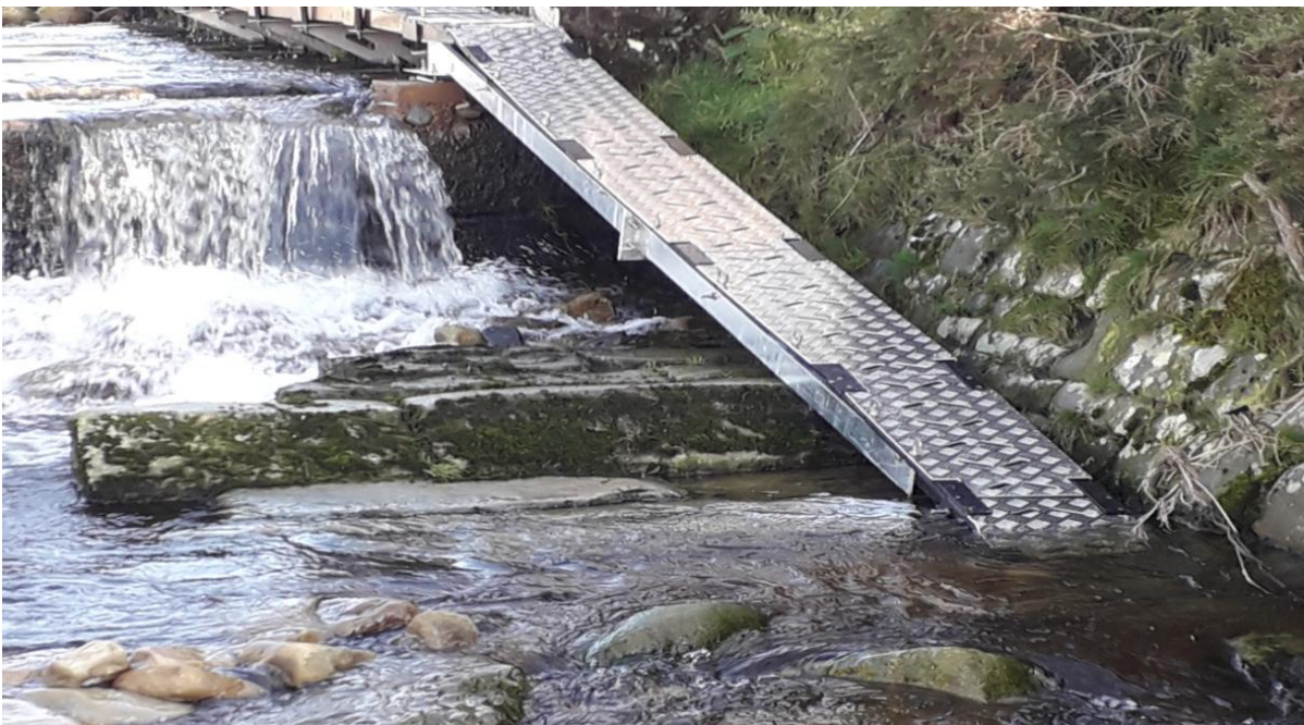
Figure 2 River Calder Intake - New eel pass
