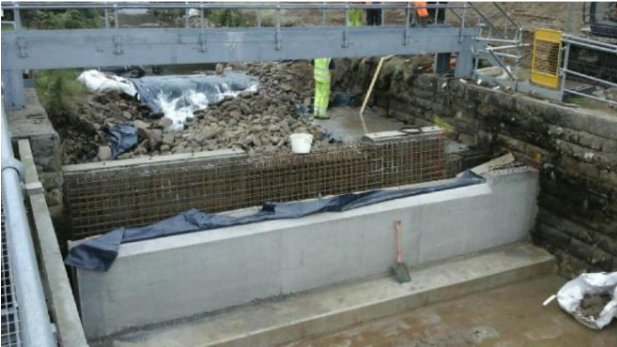
Figure 2 River Calder Intake - New eel pass
