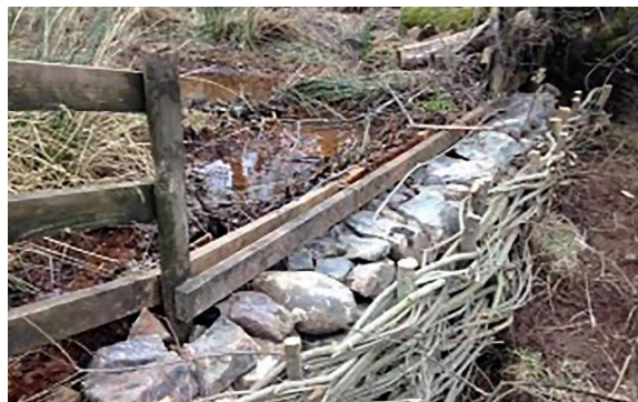
Figure 14 Example of stone wall leaky dam installed by the Project Officer to reduce runoff from an ochorous ditch in the River Ehen catchment; a number of such interventions have been installed across the catchment
