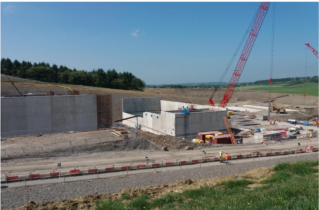
Figure 11 Construction of new Williamsgate Water Treatment Works
