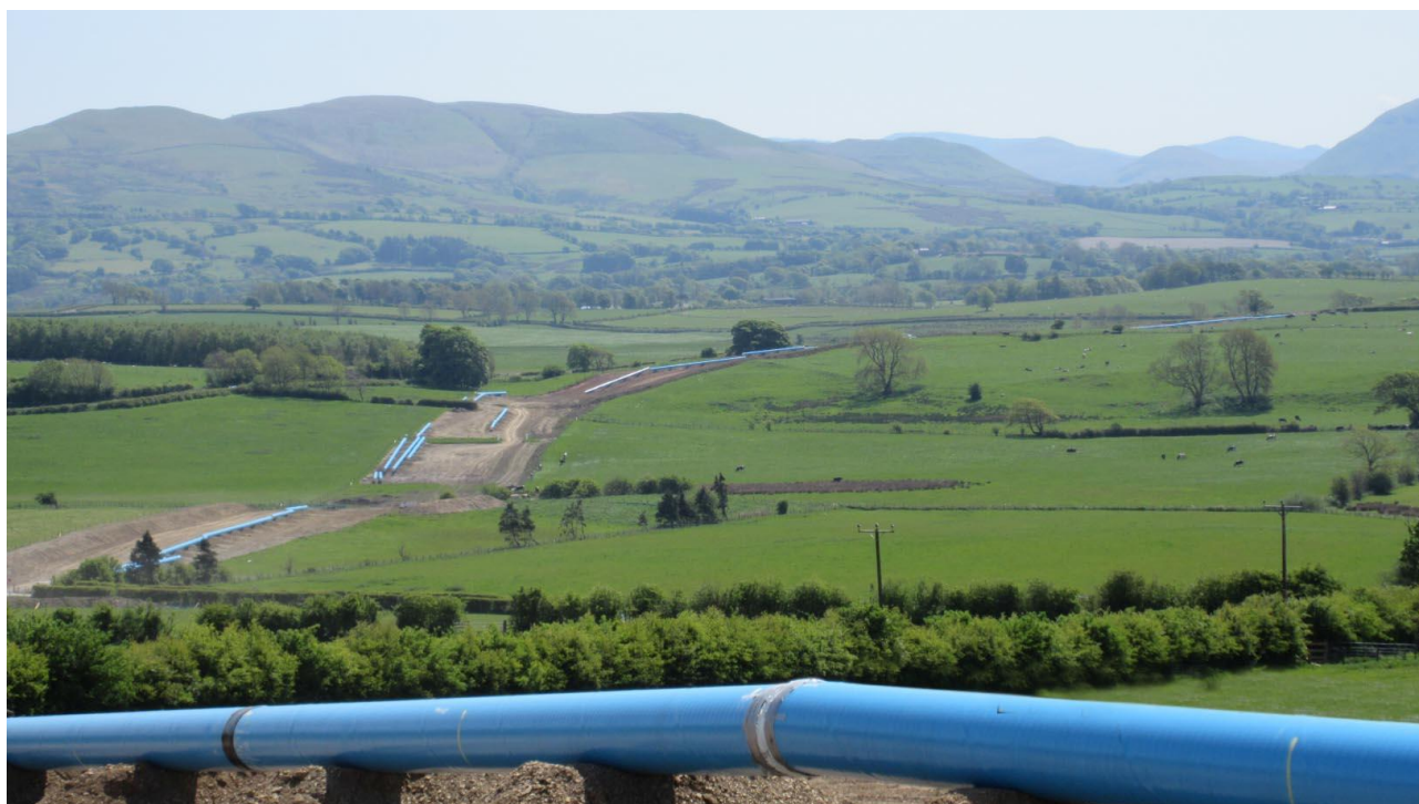
Figure 12 Construction of Thirlmere transfer water mains
