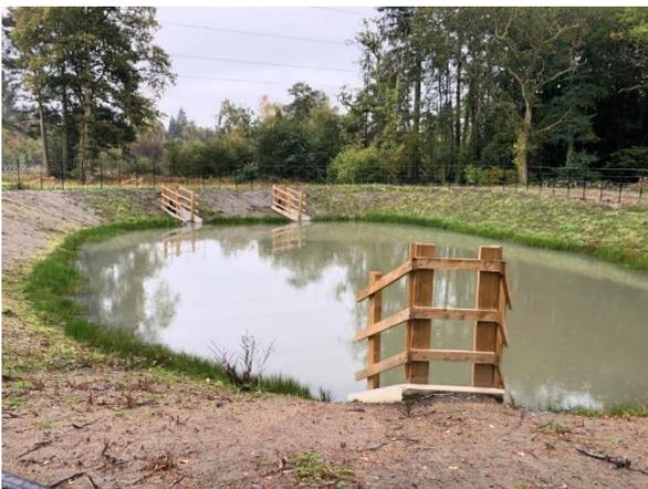
This is a sedimentation basin treating runoff from a trunk road in Devon; it was installed by Highways England and discharges to an extensive reed bed.
