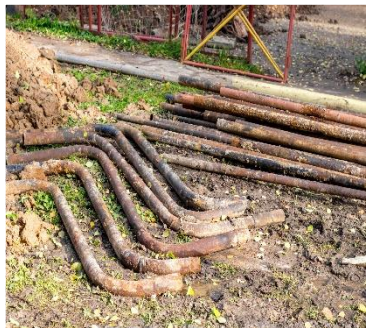
Lead pipe replacement for deprived areas
