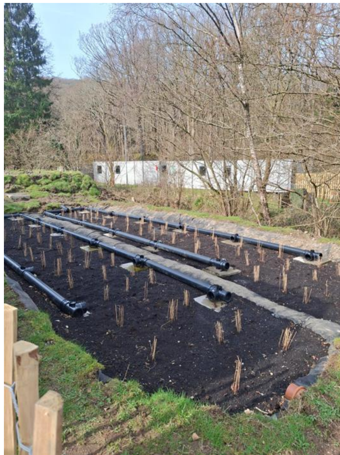
Figure 1: Picture of absorptive media bed with reeds after planting.
