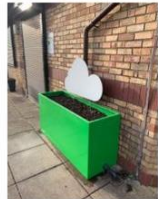
Down-pipe rain garden
