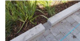
Rain garden kerb for surface water run-off
