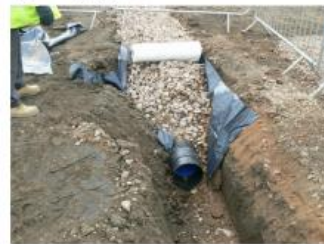
Fig 9: Installation of final filter drain
