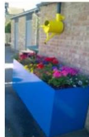
Watering can down-pipe rain garden
