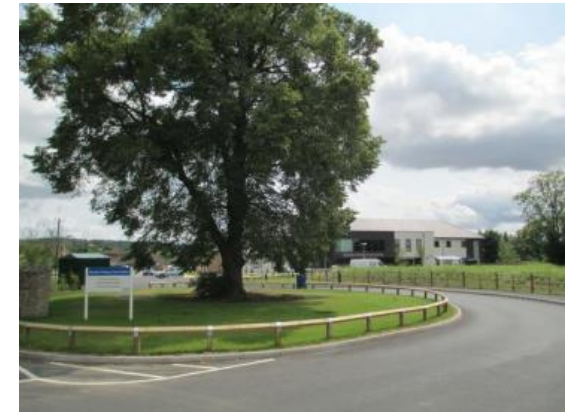
Alcester Primary Care Centre, Warwickshire ( Case study )
