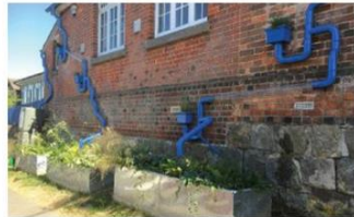
Playful downpipes and SUDS planter
