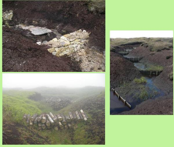
Pictures showing a variety of gully blocking techniques at Kinder catchment where around 1,800 dams are being installed to raise the water table, encourage peat sedimentation & revegetation
