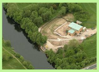
during floods and a balancing tank to allow screen washing waste to be collected and allow the pumping station to continue to operate. Ancillary works included relocating a pollution monitoring station to inside the bund and removing the old one.
