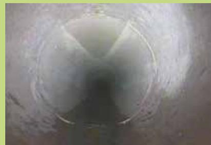
Pipe in good condition no defects or cracks, water flowing freely
