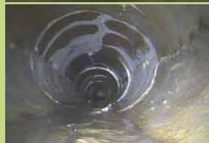
Pipe in poor condition, cracks, collapsing change in shape. This cannot be built over or near to
