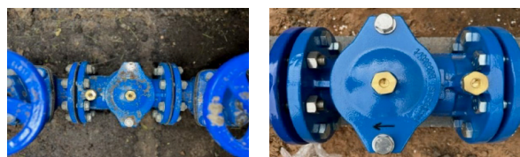
Suitably approved backflow preventer installation
