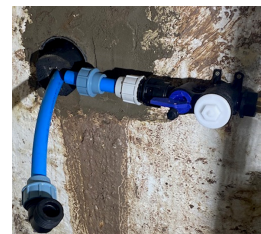
Example of a service pipe being ducted and insulated through a basement wall
