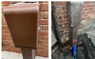
Wall mounted box together with INSUduct extension
