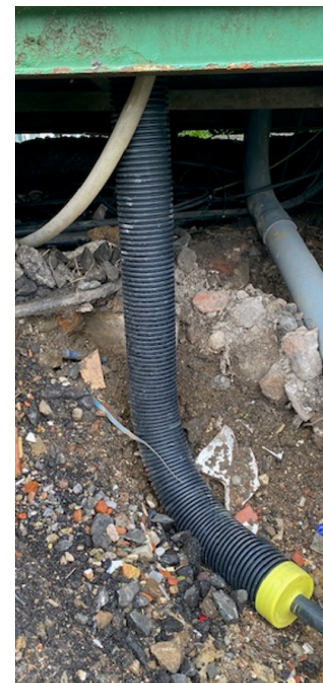
Example of a bottom entry supply prior to backfilling
