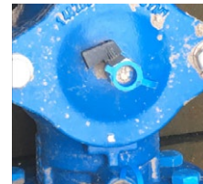
Test points on a SOCLA EA453
