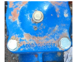
Test points blanked off on a SOCLA EA453
