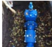
Watts Ocean FC Series backflow preventer together
