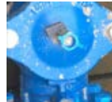
Test points on a SOCLA EA453
