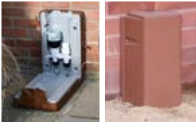
Wall mount box in situ and insuduct
