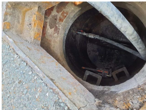
Figure 3: Grout injection to seal a manhole
