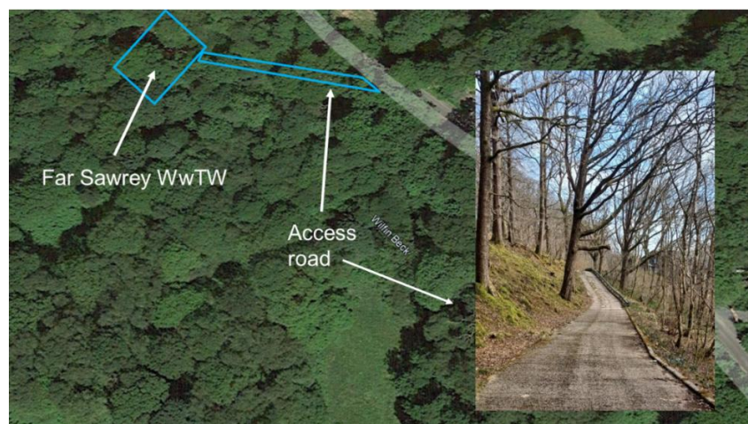
Figure 2: Location and access to Far Sawrey WwTW
