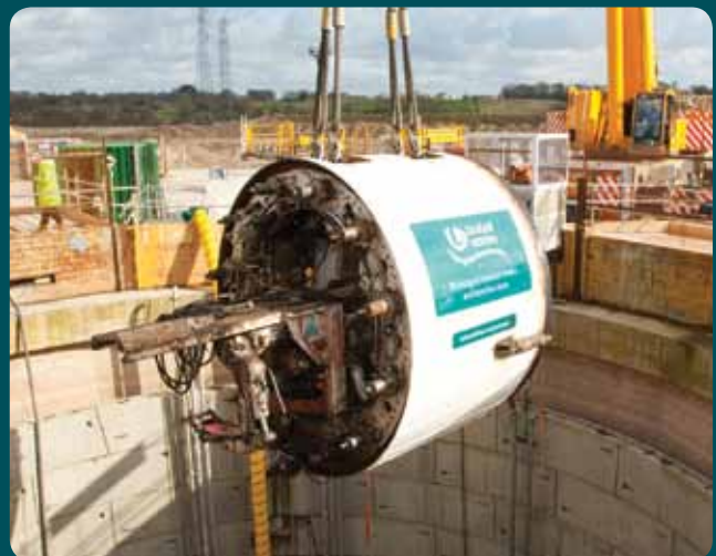
Pictured: Tunnelling work on a £160 million environmental improvement scheme in Preston.
