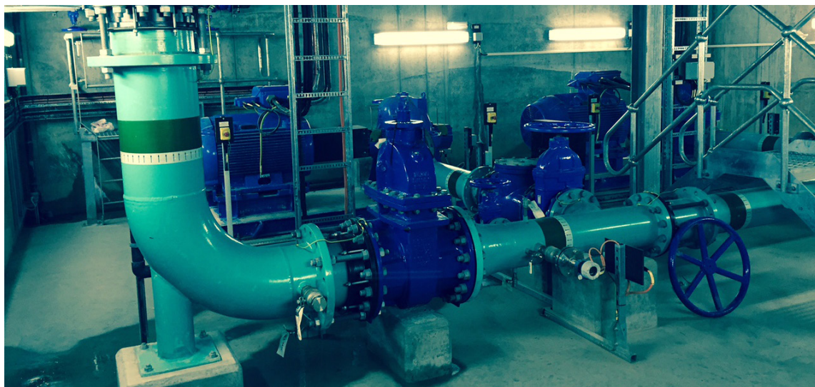
Figure 1 The completed South Egremont scheme pumping station at Gullely Flatts which transfers untreated borehole water to Ennerdale WTW
