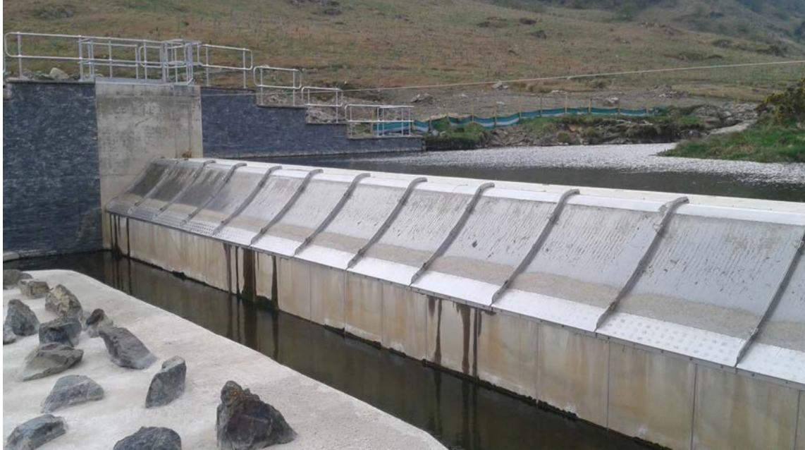
Figure 2 Swindale Beck intake following modifications to deliver sustainability changes
