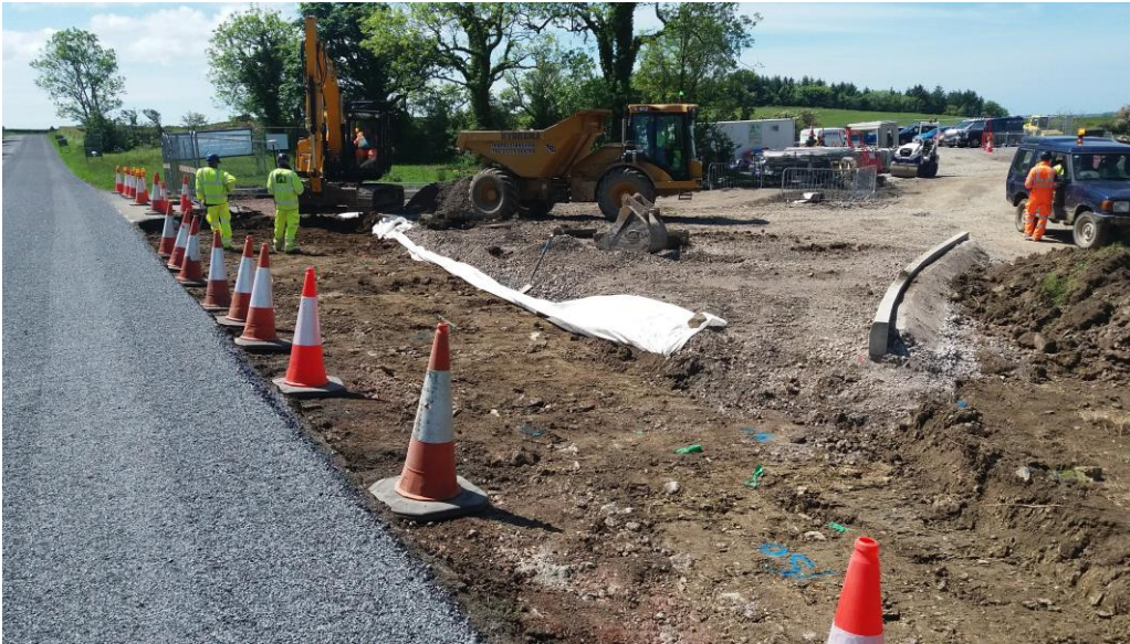
Figure 13 Site of planned new Williamsgate Water Treatment Works
