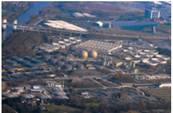
Top: Davyhulme WwTW in 2015
